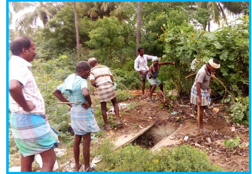
OfERR construction consultant Mrs. Caryll Toser inspecting the Government Toilet Cluster in Thillavidangal village which needed repairs & instructing OfERR staff and village leaders on the repairs to be carried out. Following which OfERR staff galvanized the Village people to clean the septic tank before embarking on repairs
